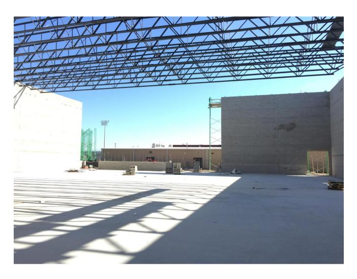
**STRUCTURAL** – Steel roof joists are being lifted and welded into place at the Main Gymnasium. Erection of the block walls continue on the east wall of the gymnasium.
