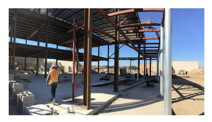
STEEL STRUCTURE - Roof decking and floor decking have been welded in place at the three story steel structure in the background and at the Large Group Instruction (LGI) Room in the foreground.
