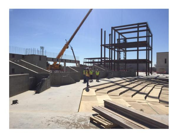
**PERFORMING ARTS CENTER** – The stepped seating area in front of the stage is on the right. The seating area to the left will be 2<sup>nd</sup> level seating accessible through stairs and an elevator. Beyond is the erection of the three story classroom building structure in progress.
